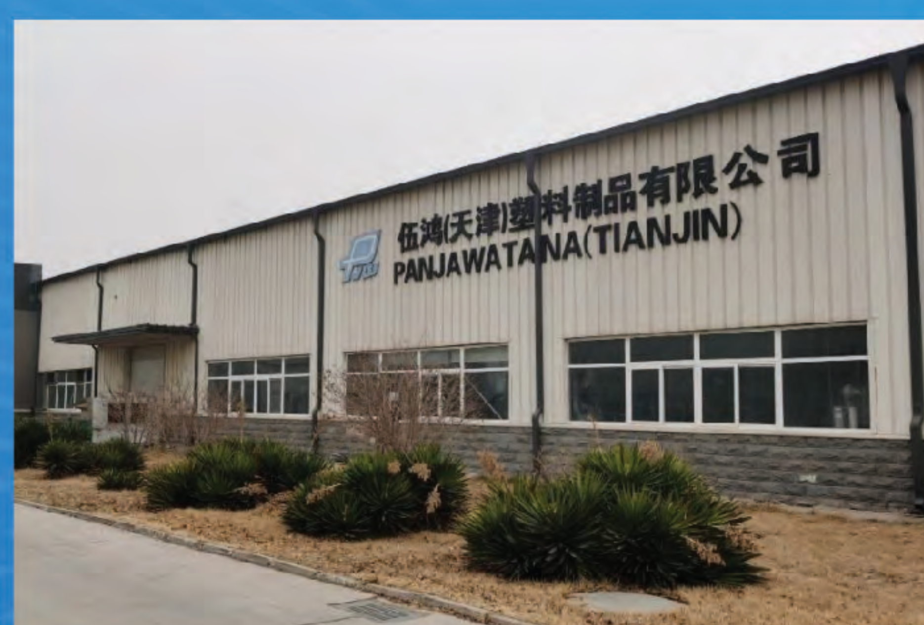
Tianjin Branch , China
